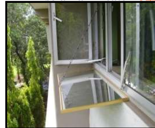
Day light retrofit
